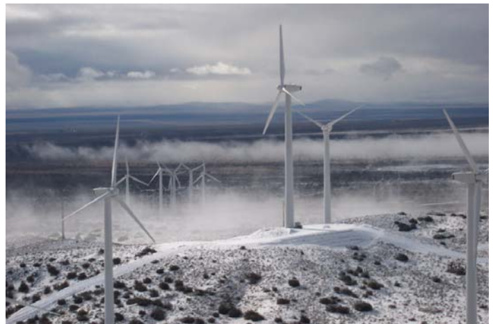
System 3 Inc. worked on the Oasis Wind Farm in Tehachapi, California.
